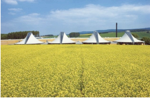
Famous symbol for employees and social orientation at Wilkhahn: The production pavilion designed by architect Frei Otto
