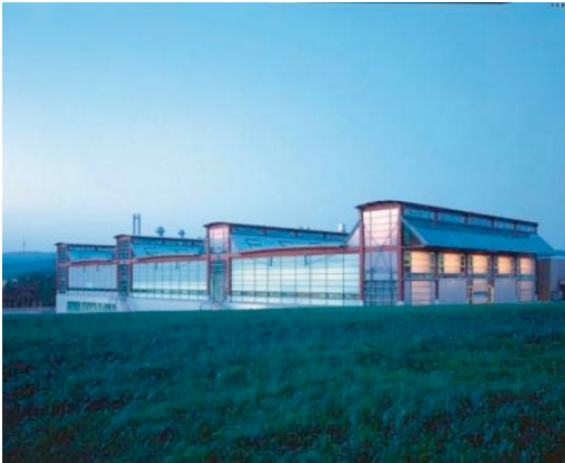
The production halls, built according to plans by architect Professor Thomas Herzog, stand for the consistent realization of a "green roof", utilization of daylight and the use of the renewable raw material of wood as a key building component. These halls are regarded as a model of excellence for ecologically focused industrial architecture. Photo: Wilkhahn
